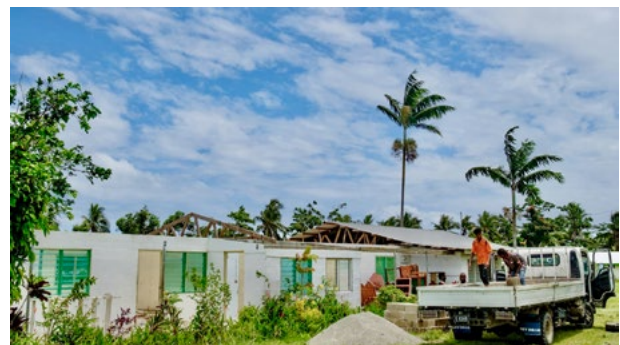
Repairing a staff house
