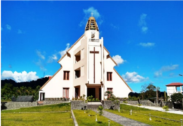
Same Presbyterian Church building
